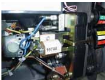
MOC with Motor Operator
