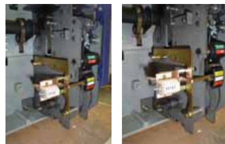
MOC without Motor Operator
